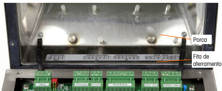
Figura 3-11: Soltar as fitas de aterramento
