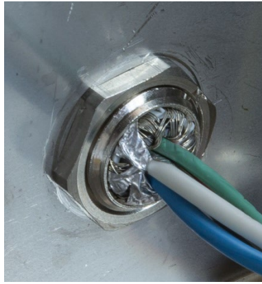
Figure A-58: Cable Gland Nut Installed
